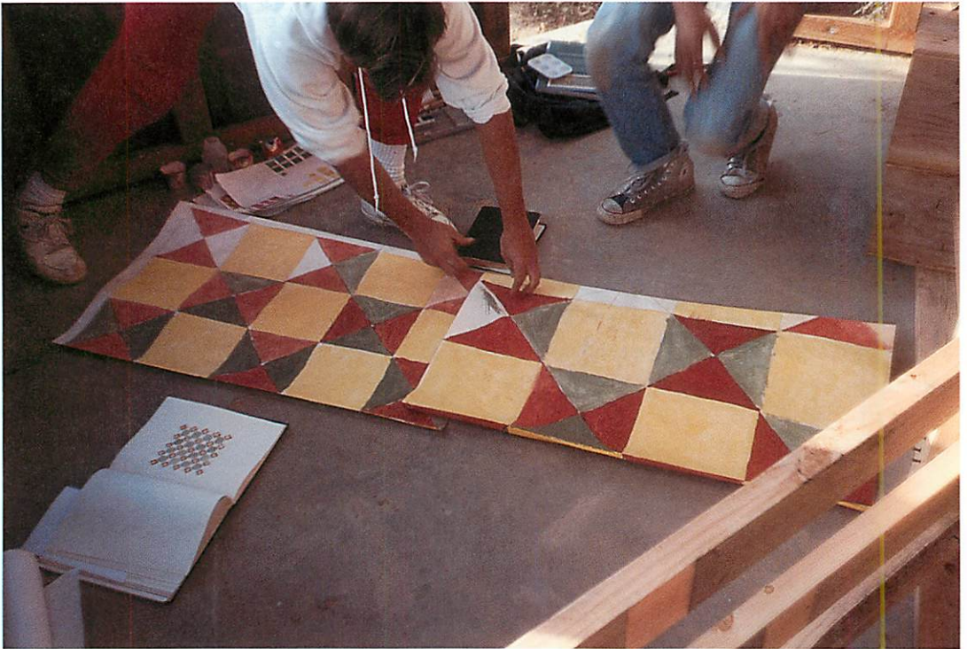
Three colored mockups on butcher's paper, to try on the floor of the actual room in order to determine the best scale for the floor pattern
