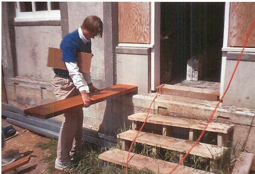
Using a simple board to judge the height, width, and length of a concrete parapet which was to be built on both sides of the concrete front door steps
