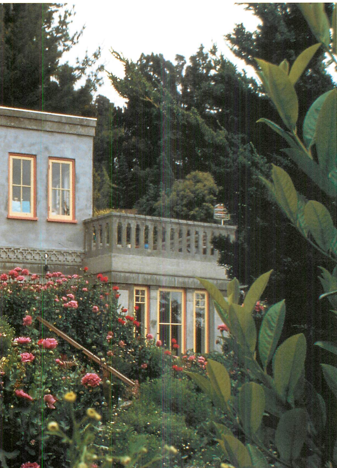
The finished house
