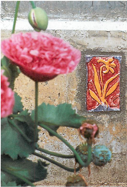
A lily-tile in the stem wall of the foundation
