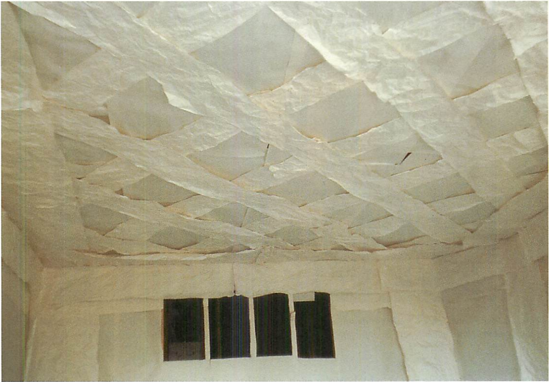
Another view, looking at the middle of the ceiling
