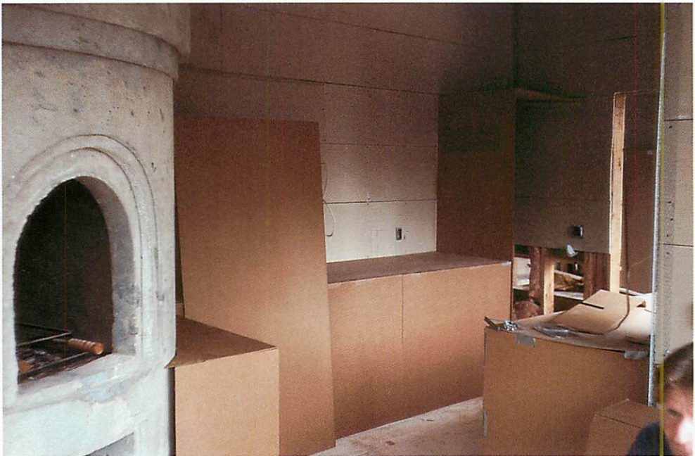
The kitchen mocked up in its entirety in cardboard, so we could see just how to make the kitchen fireplace. The idea of a cylinder had already occurred to me from seeing the room shape and recognizing its two lines of sight. Now we had to make the cylinder work, and to do that we had to have the full three-dimensional configuration, as it was going to be. We had to make many many versions before it all sat right.
