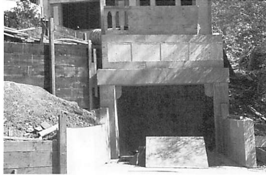
Formwork on the massive concrete brackets which frame the garage
